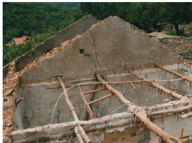
Figures 10, 11. Photographs taken during the renovation of the Yu Zhenli Studio, 2008.
